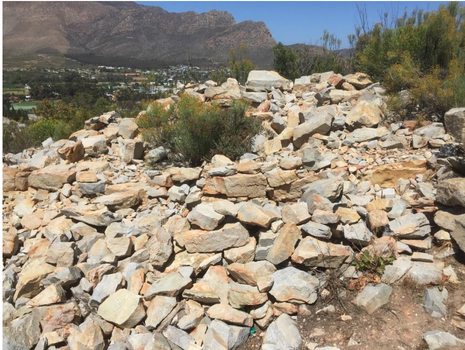
Bergsig 2021 Sadly this site has been badly vandalised
