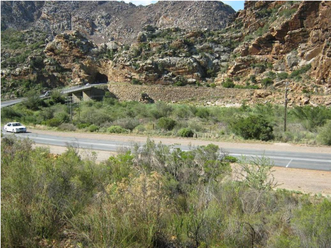
View eastwards towards the rock tunnel with the fort perched on the rocks above
