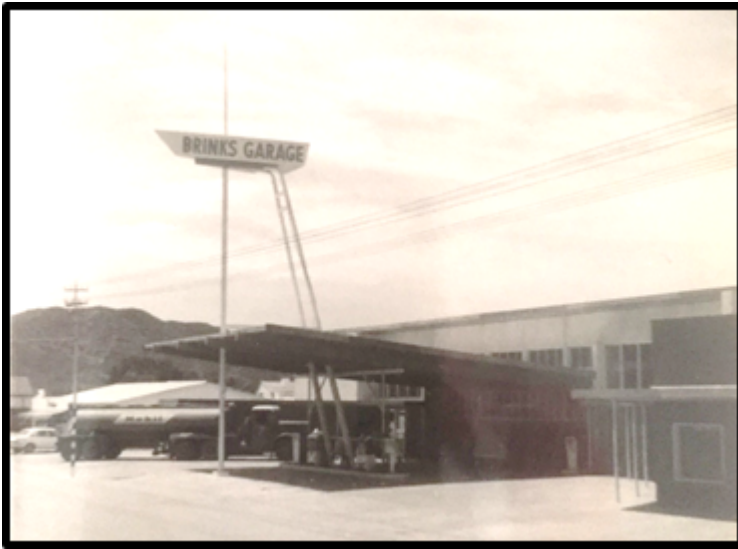
Brinks Garage Bath Street
