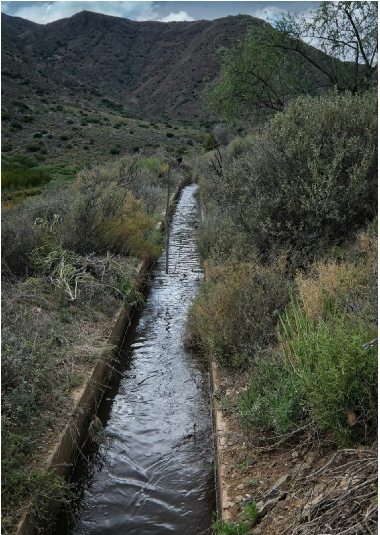
All sections of canal still in use are extremely well maintained
