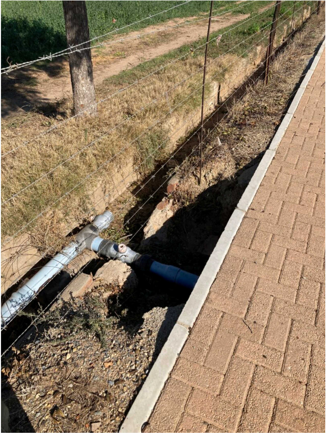
Crossing under Long Street. The blue pipes were not part of the original scheme.
