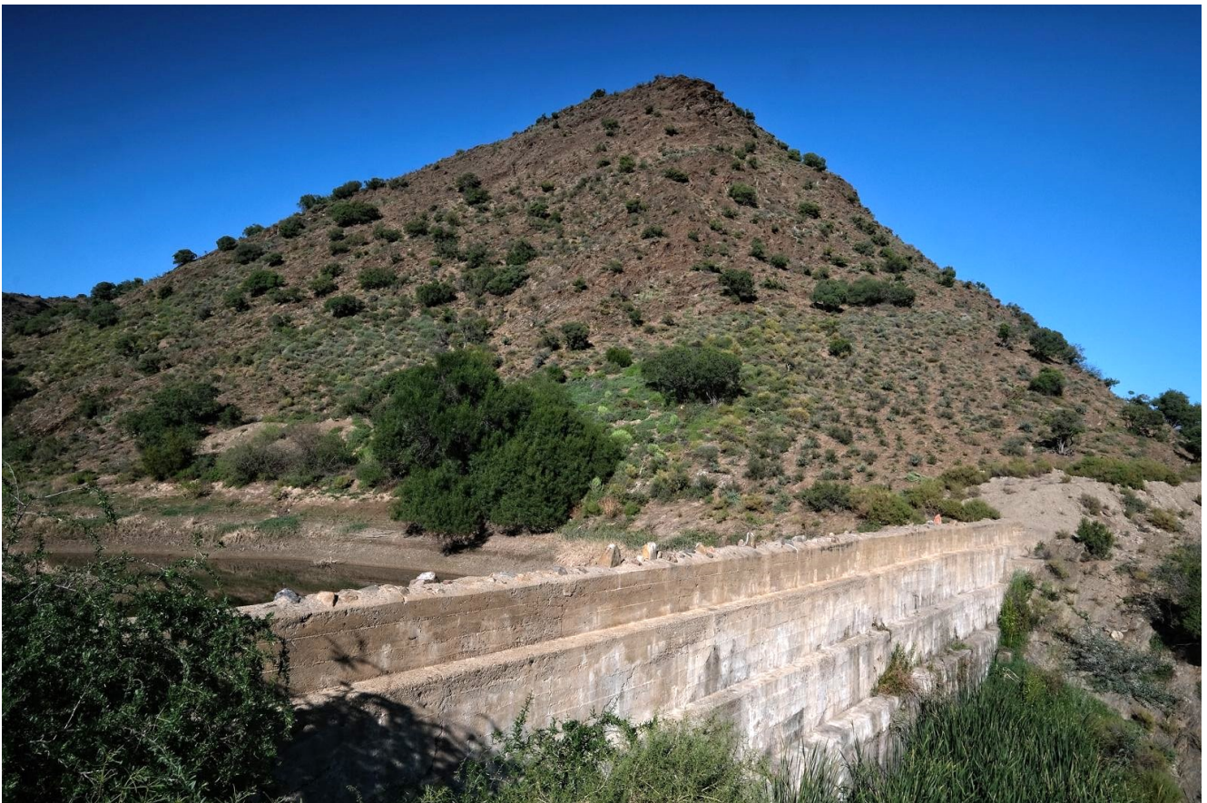
One of the storage dams in the leiwat canal
