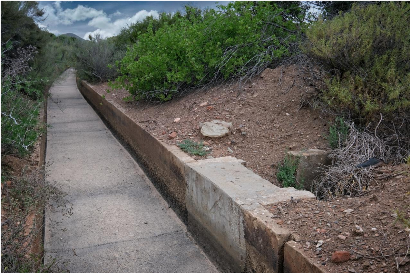
A disused sluiceway
