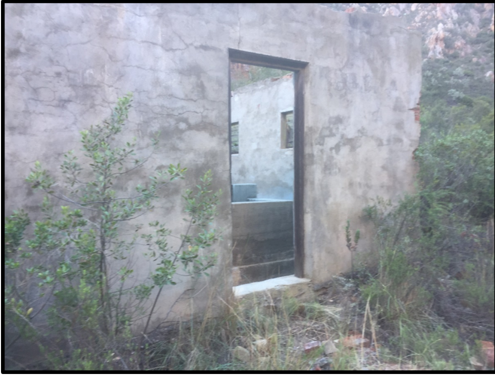
The old building housing the filtration plant
