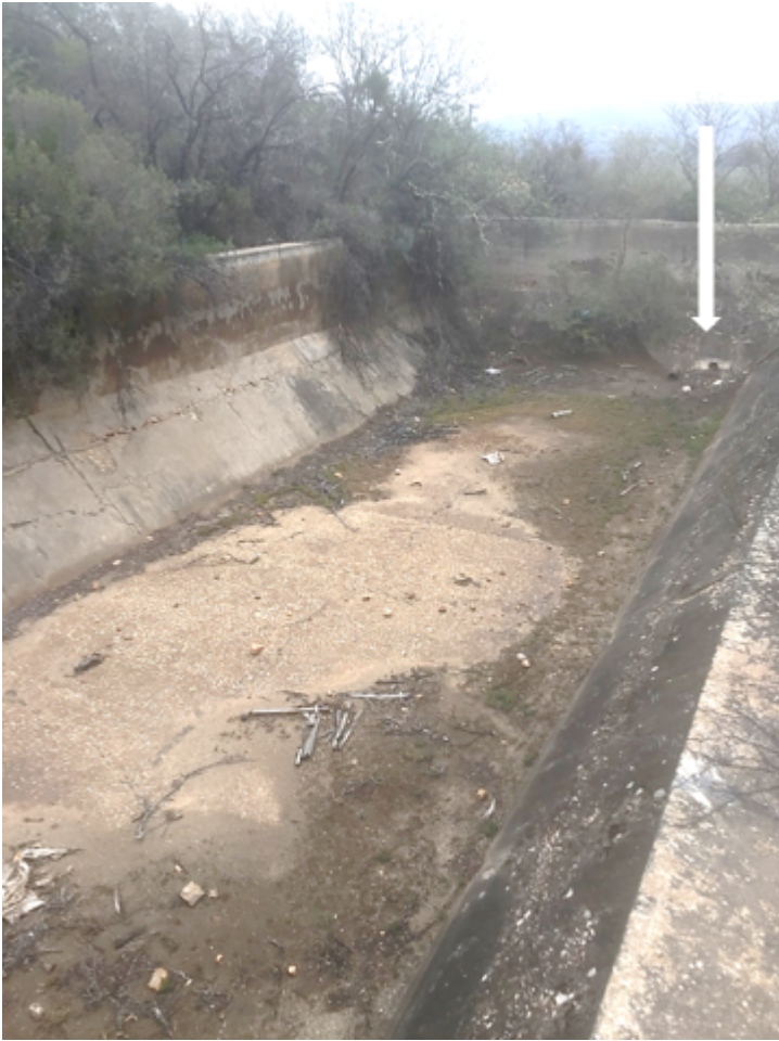
Arrow indicates outlet pipes
