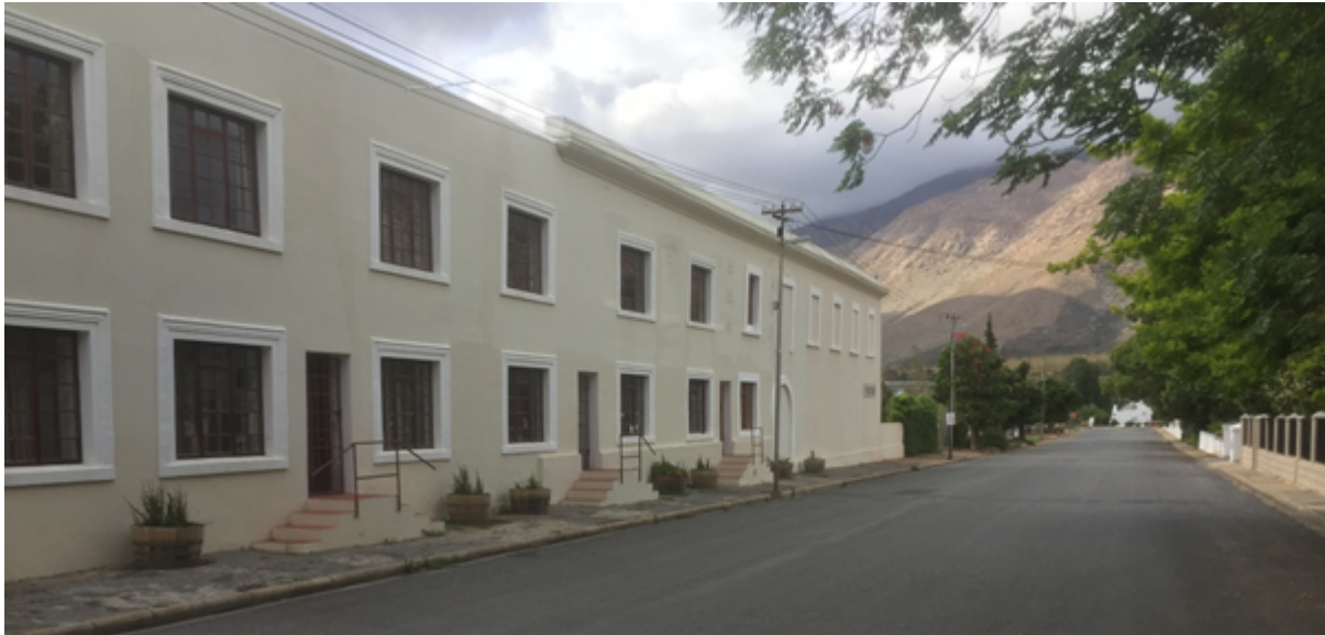
The old company cold rooms converted into living accommodation. (2019)
