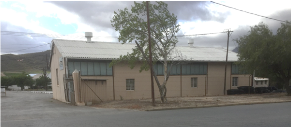
The group workshop building (2019)
